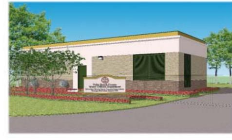
Designed for the Belvedere/Westgate CRA and PBC Water Utility Department, the project consist of a vacuum wastewater collection and effluent pump building to serve the Belvedere/Westgate Community. The building has also been designed to withstand a Category 5 hurricane, with basic wind speed at 190 MPG. Construction is expected to finish by the end of 2012.
