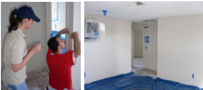
Elena Contreras takes notes as Jon Swergold measures the wall for the chair rail. The apartment is prepped and ready for painting with the fixtures and windows taped and a tarp covering the floor.
